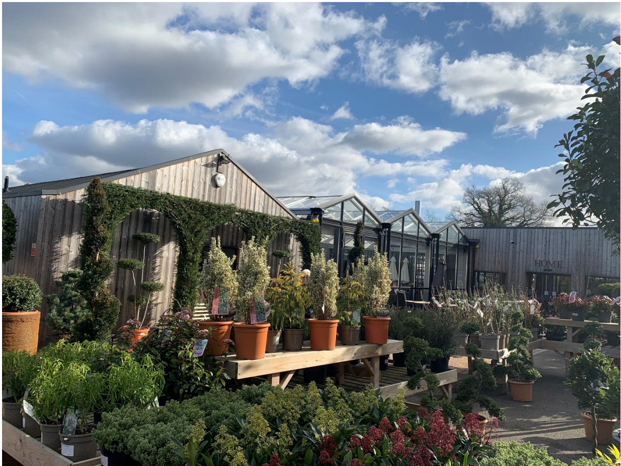
Elevation of glass house extension
