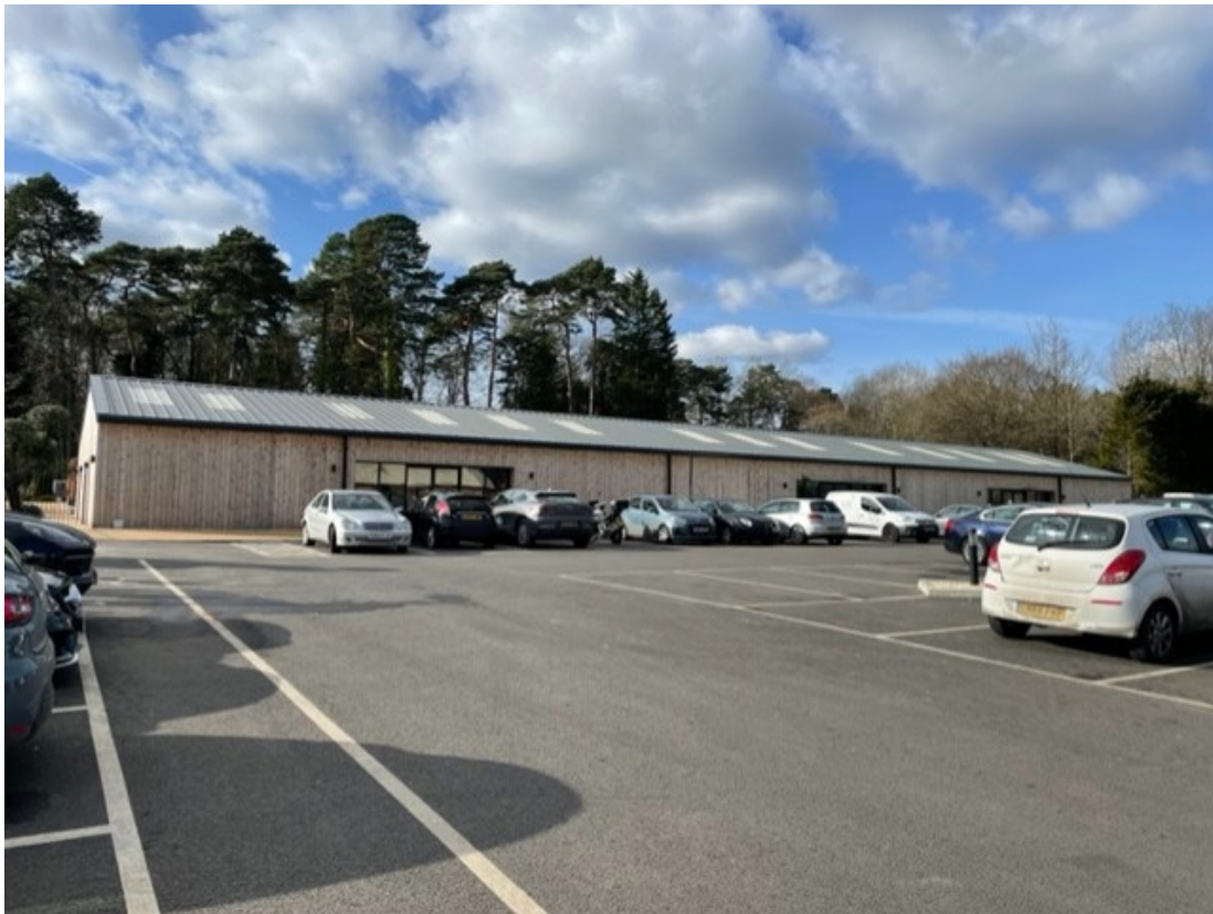
Front elevation and car park
