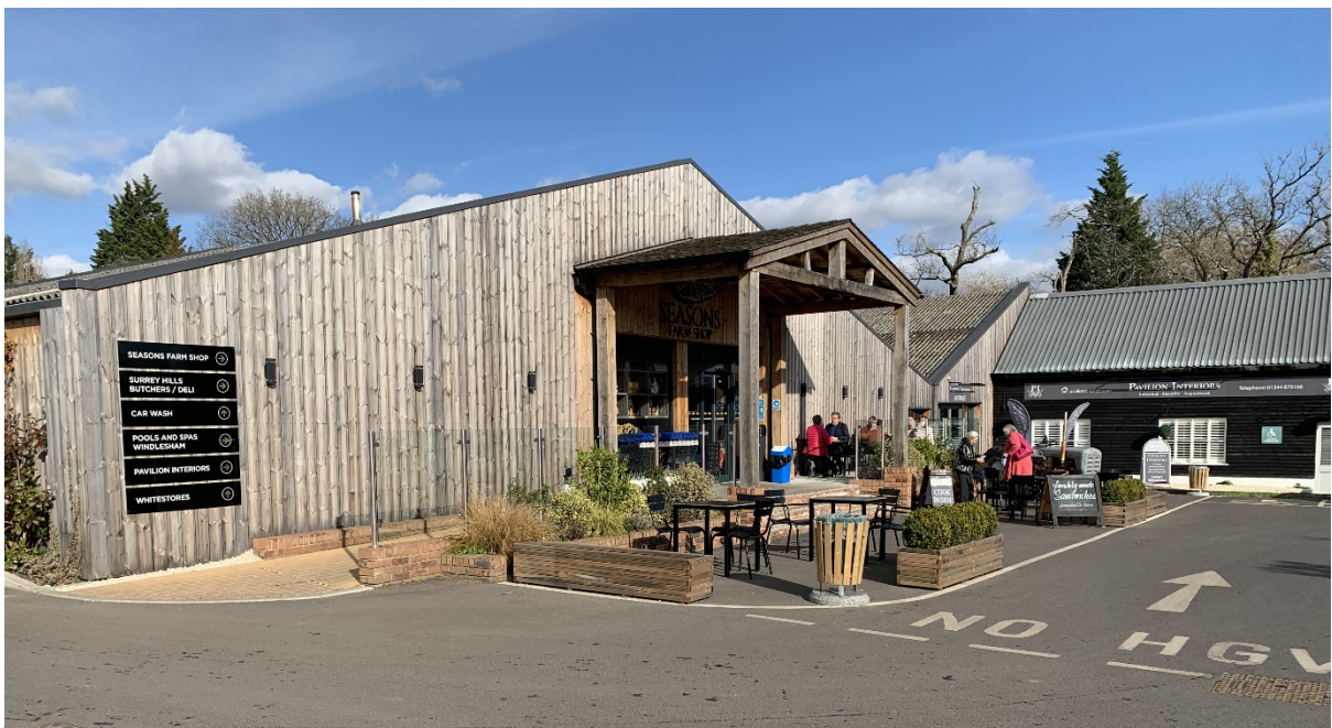
Front elevation Seasons Farm Shop
